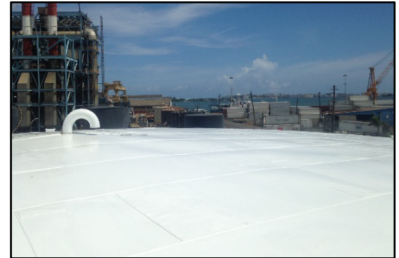
After: Finished repairs and top coated external of tank roof.
